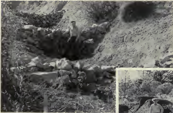
SAVING THE SOIL —at left, three rock check dams constructed from material available at the site, hold back streams that run rampant after heavy rains. Below, brush check dams which retain material washed down the gullies. Both are vital parts of the erosion control program in the Keswick reservoir and watershed area. Photos by J. D. Leeper, Region 2, photographer.
